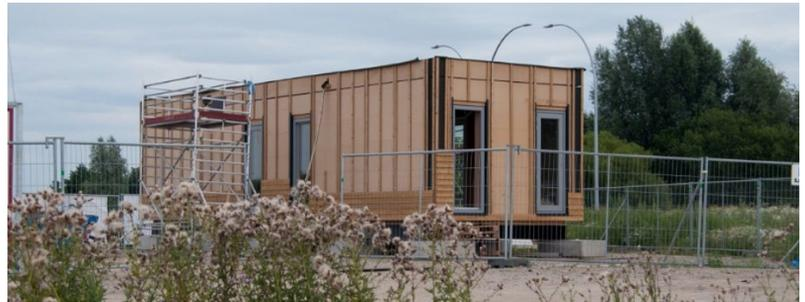
design of the house allows users to disconnect panels or to expand the frame. Circularity is seen with recycled materials, insulation made from biomass and wood as a substitute for concrete. Even amidst COVID-19, Team Celcius succeeded in creating a product that can inspire the future of the Dutch housing market.
